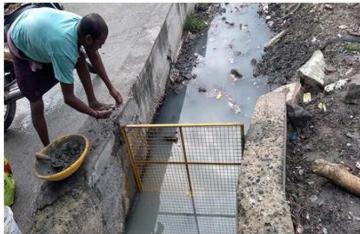
Screening mesh placed at one of the spots
